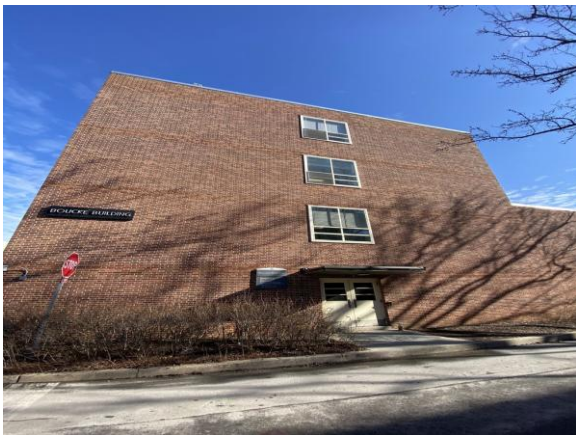
0013-000039a 1/30/2025 Brick facade and glazing Exterior
