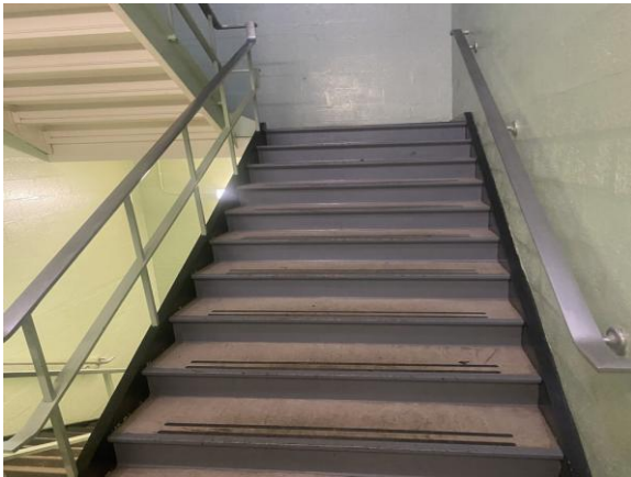
0013-000010a 1/30/2025 CMU, concrete treads, and metal railing Stairwell
