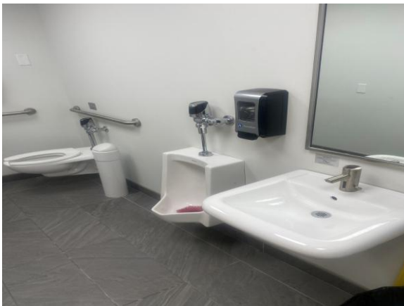
0013-000027a 1/30/2025 Finished walls, tile flooring, accessible water closet, urinal, and lavatory Restroom
