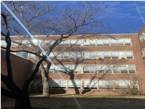
0013-000038a 1/30/2025 Brick facade and glazing Exterior
