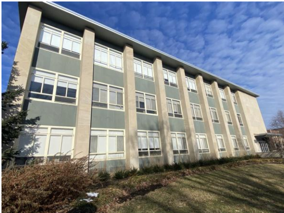
0013-000035a 1/30/2025 Granite panels, attached columns, and glazing Exterior
