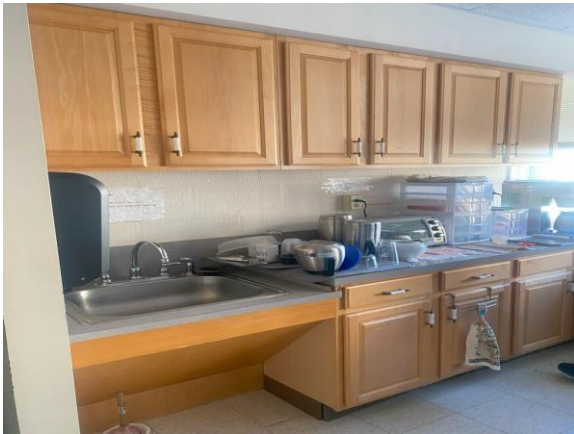
0013-000022a 1/30/2025 Acoustical ceiling tile, vinyl composite tile, and casework with a sink Break Area
