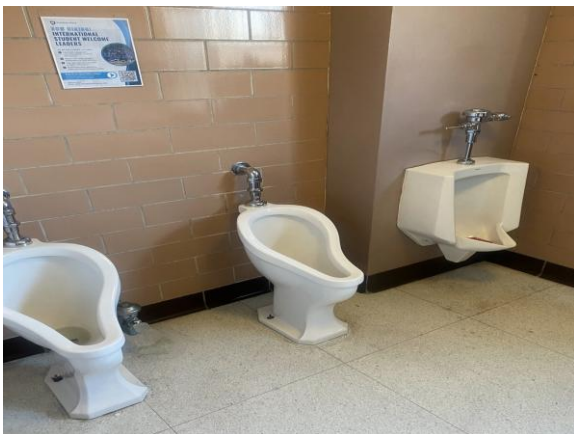
0013-000015a 1/30/2025 Glazed brick, terrazzo, and floor and wall-hung urinals Restroom
