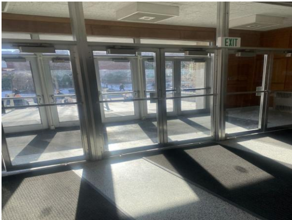
0013-000032a 1/30/2025 Metal and glass interior entry doors Entrance
