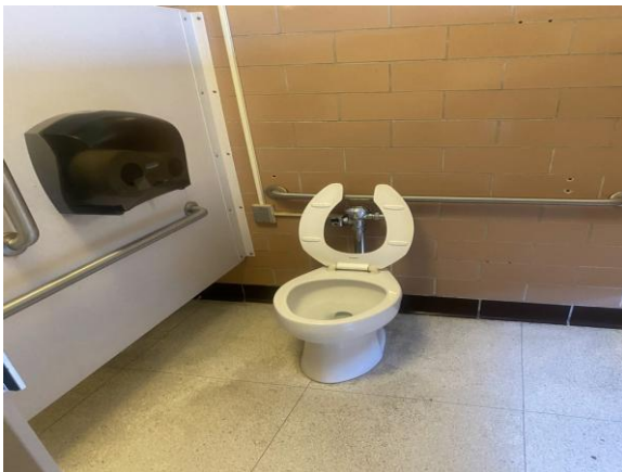
0013-000012a 1/30/2025 Glazed brick, terrazzo, and accessible water closet Restroom
