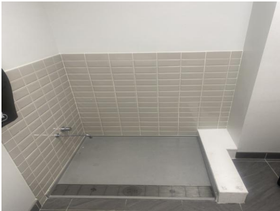
0013-000026a 1/30/2025 Tile walls and floor Foot bath
