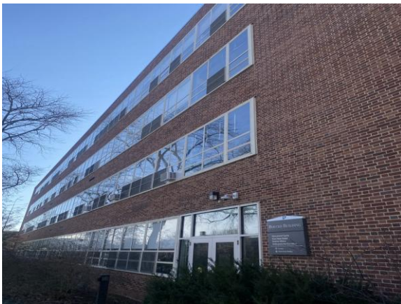
0013-000042a 1/30/2025 Brick facade, glazing, and metal and glass entry doors Exterior
