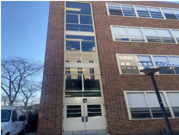
0013-000041a 1/30/2025 Brick facade, glazing, and hollow-metal entry doors Exterior
