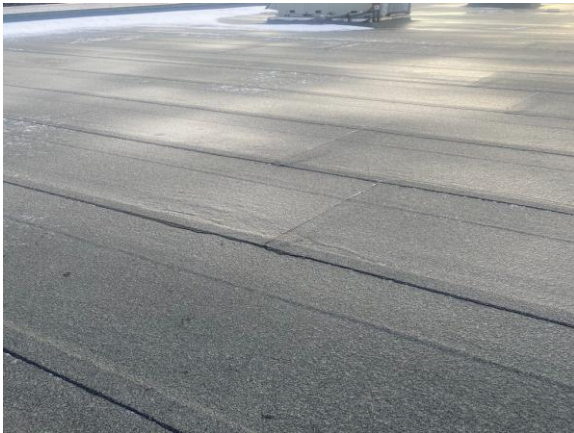
0013-000005a 1/30/2025 Modified bitumen roof Roof
