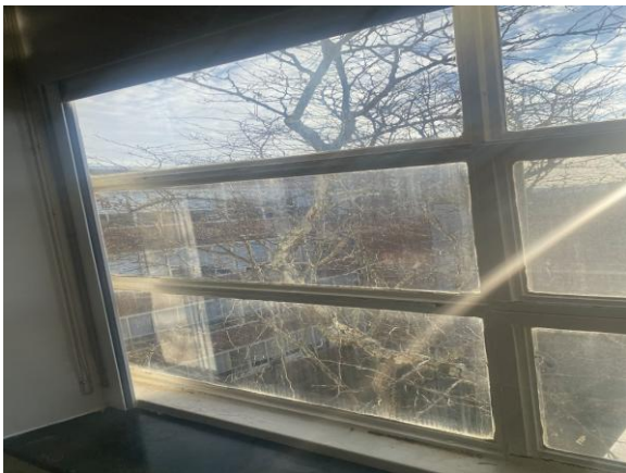
0013-000021a 1/30/2025 Single-pane windows Classroom
