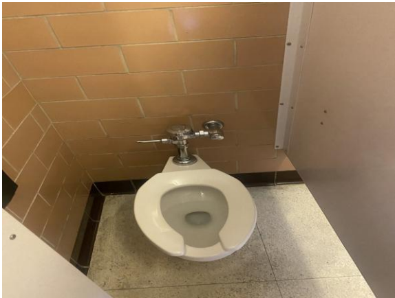
0013-000013a 1/30/2025 Glazed brick, terrazzo, and tankless water closet Restroom
