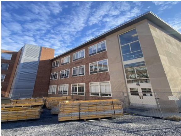
0013-000037a 1/30/2025 Concrete panels, brick facade, and glazing Exterior
