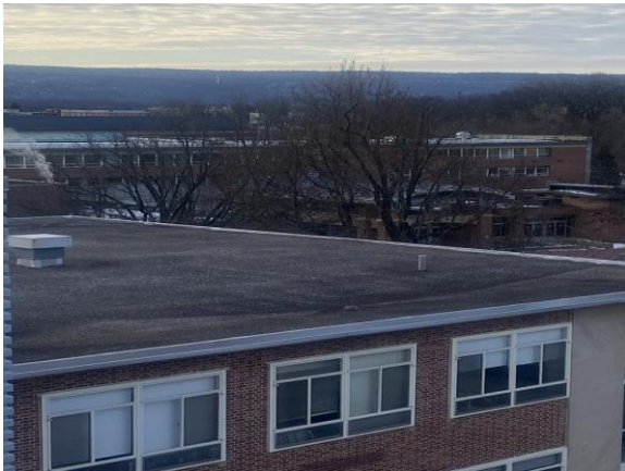
0013-000008a 1/30/2025 Built-up ballasted roof Lower roof
