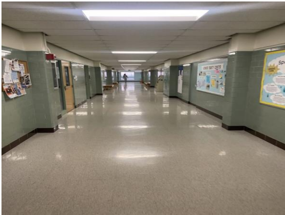
0013-000031a 1/30/2025 Acoustical ceiling tile, vinyl tile, and glazed brick Corridor
