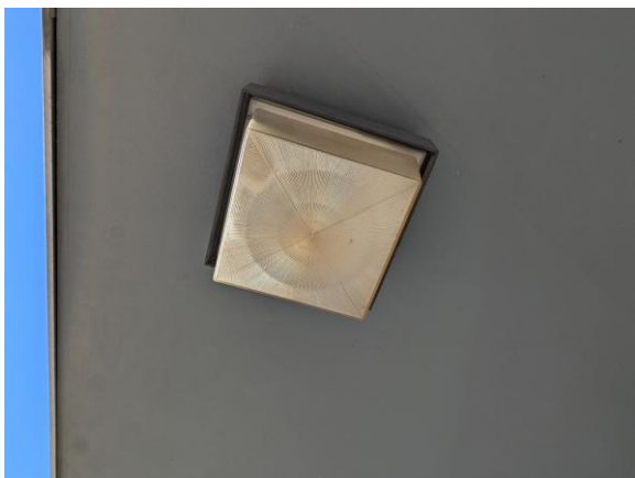
0013-000047e 1/30/2025 Surface-mounted HID fixture East elevation
