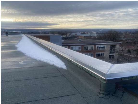
0013-000007a 1/30/2025 Modified bitumen roof Roof
