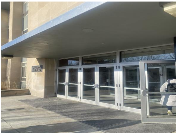
0013-000033a 1/30/2025 Metal and glass exterior entry doors Entrance
