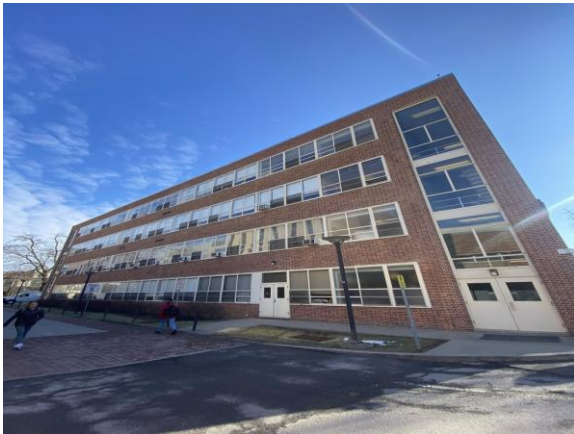
0013-000040a 1/30/2025 Brick facade, glazing, and hollow-metal entry doors Exterior
