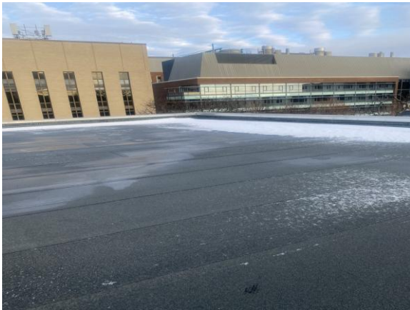
0013-000004a 1/30/2025 Modified bitumen roof Roof
