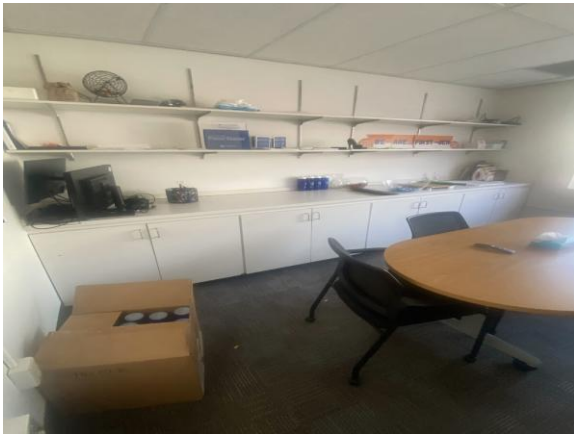
0013-000028a 1/30/2025 2x4 acoustical ceiling tile, carpet, finished walls, and casework Work room
