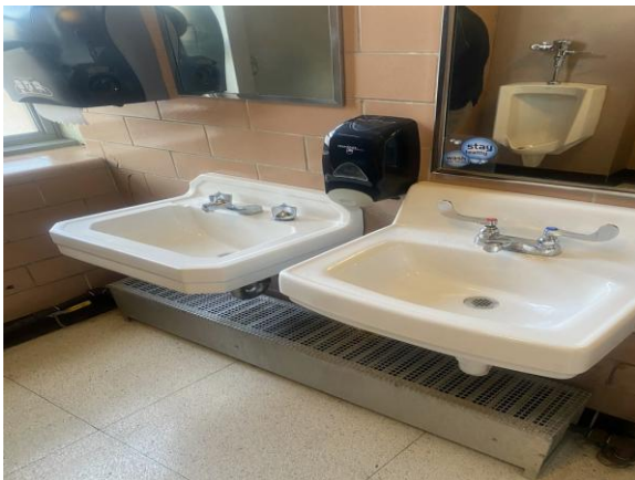
0013-000014a 1/30/2025 Glazed brick, terrazzo, and wall-hung lavatories Restroom
