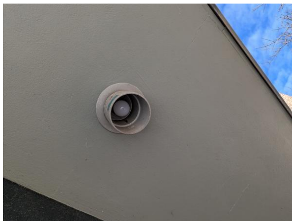
0013-000048e 1/30/2025 Can light with incandescent lamp East elevation
