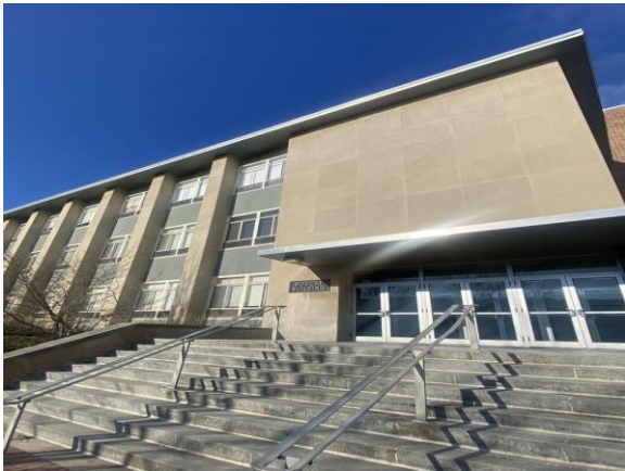
0013-000034a 1/30/2025 Concrete panels and attached columns, glazing, entry doors, and steps Exterior
