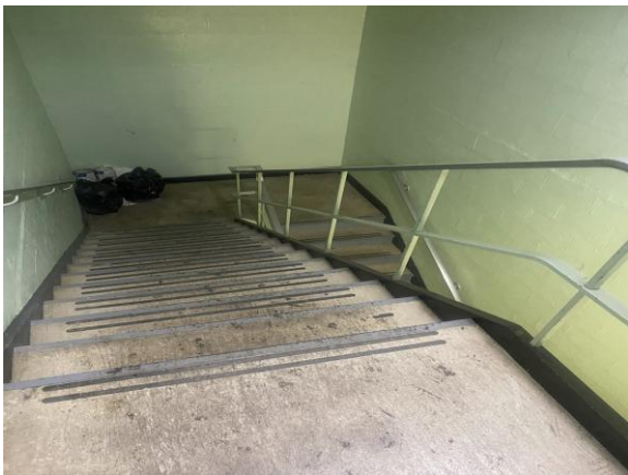
0013-000009a 1/30/2025 CMU, concrete treads and landings, and metal railing Stairwell
