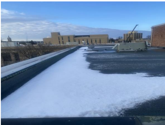
0013-000006a 1/30/2025 Modified bitumen roof Roof
