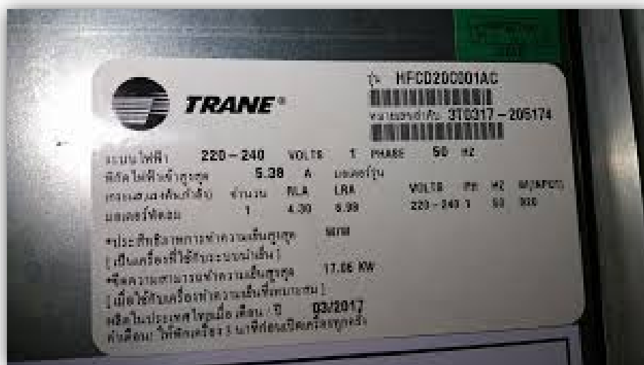
Figure 24: Name Plate Examples (Unacceptable)
