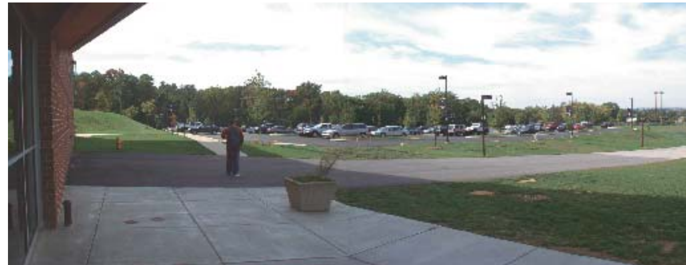
4 - Library approach from parking lot
