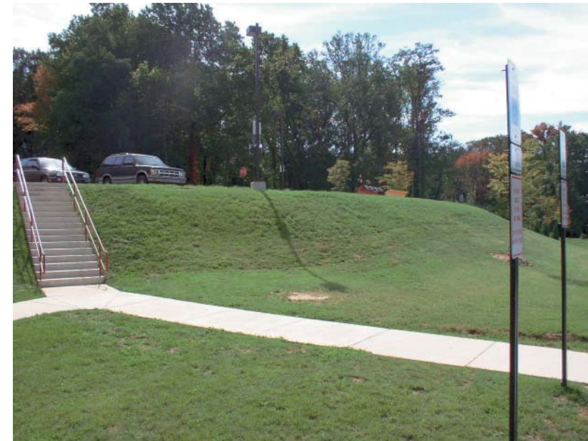
2 - Slope at service area / loading dock
