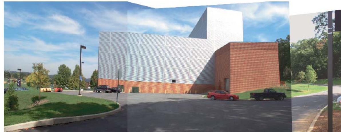
1 - Pullo Center / Library from entrance drive
