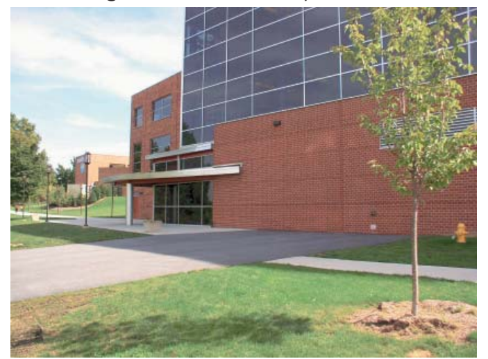
2 - Existing View of Library Entrance
