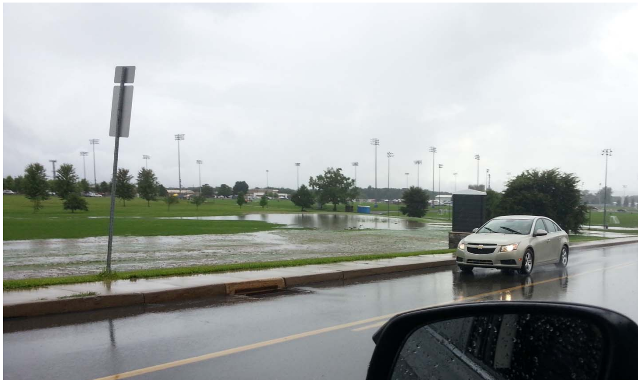
Figure 7.g. Flooding of Park Avenue from a New Stormwater Volume BMP Failure Section 7-7
