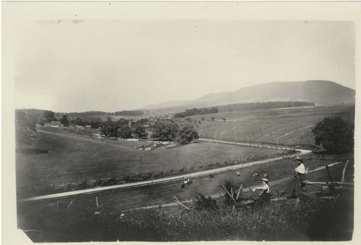
Figure 2.b. Thompson Valley Looking Over Current WWTP Site in 1890s with Thompson Spring in the Foreground.
