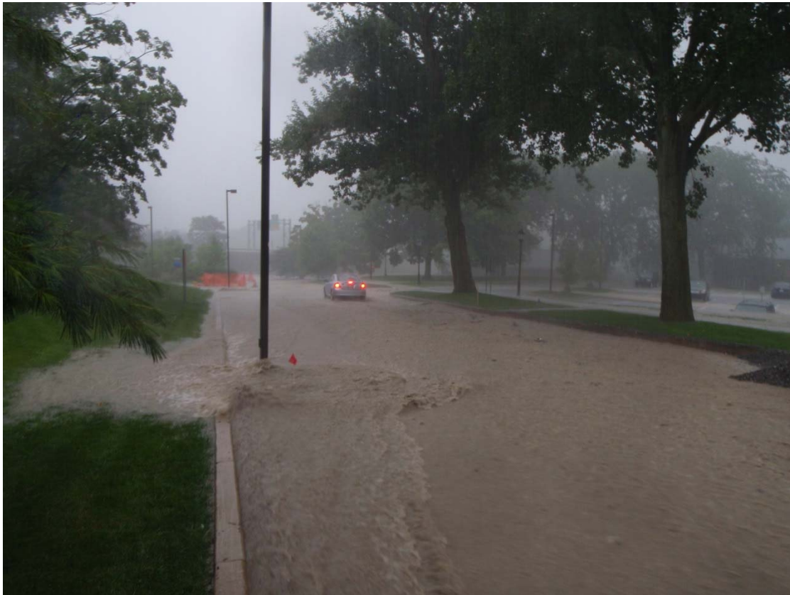
Figure 4.j. Flooding of Lower Bigler Road
