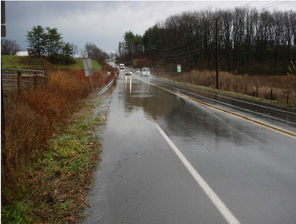
Figure 7.j. Flooding at the Sag in Fox Hollow Road During Overflow Conditions
