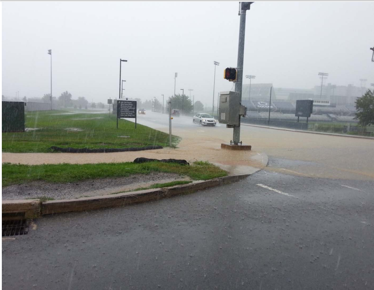
Figure 7.f. Flooding by Uncontrolled Drainage at the Intersection of Park Ave and University Dr
