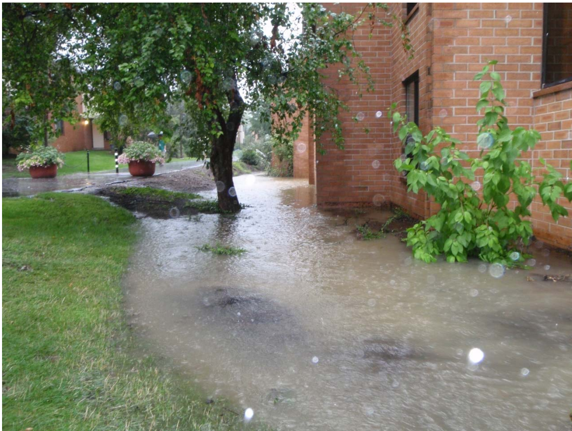
Figure 6.w. Flooding Along the North Side of Nittany 60
