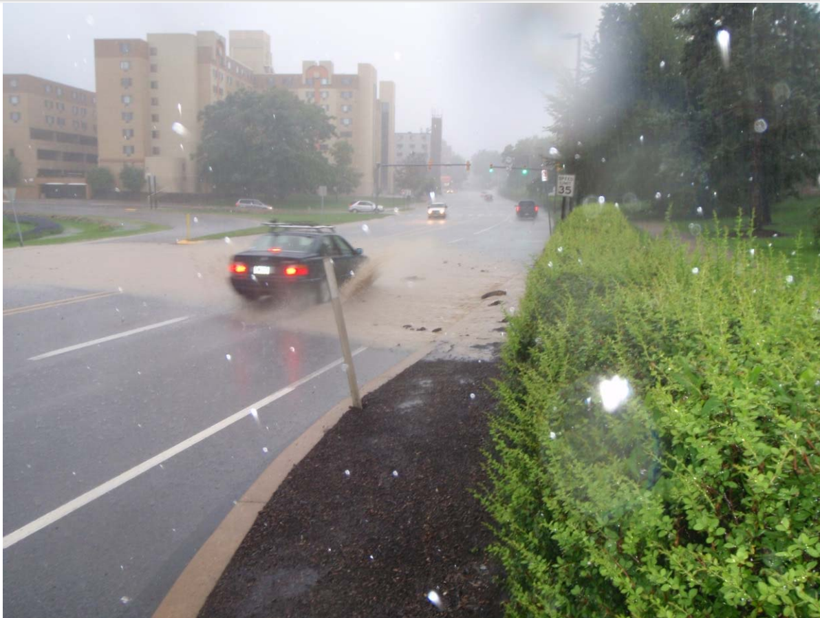
Figure 6.e. Flooding of College Ave at the University Cloverleaf from Bigler Road Runoff
