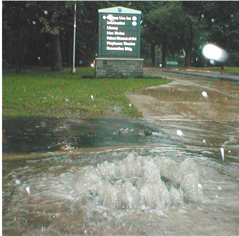
Figure 7.e. Surcharging at STMH125 along Park Avenue
