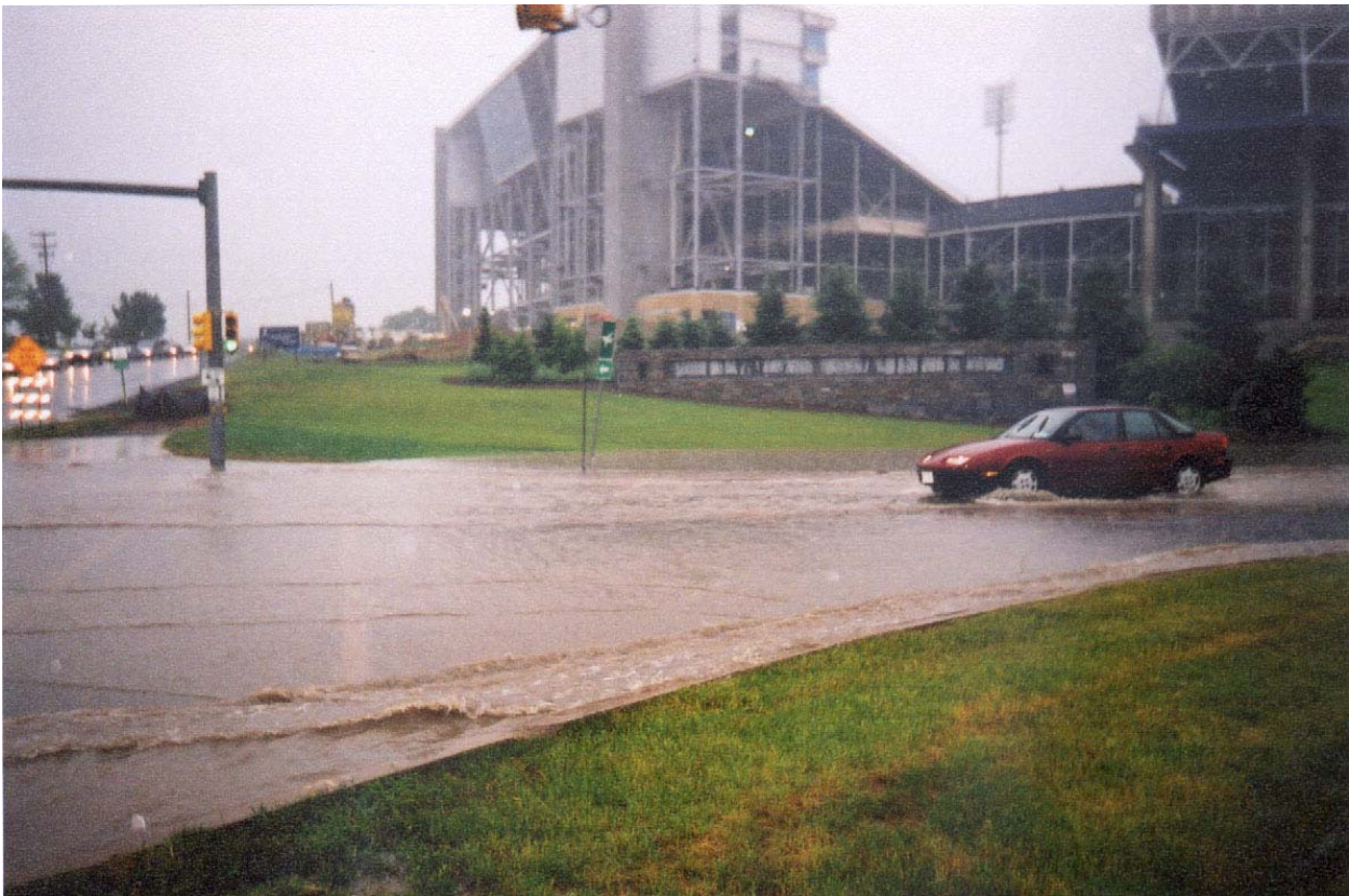
Figure 4.h. Flooding of the Intersection of Fox Hollow Road and Park Avenue
