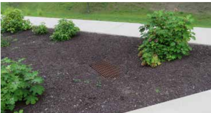
4. Mulch washes into inlets and clogs storm-water pipes
