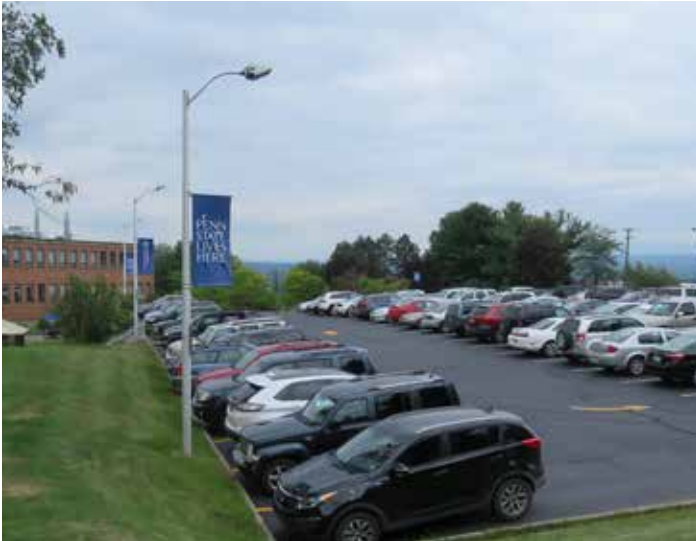
Non-standard parking lot light fixtures at Dawson parking lot
