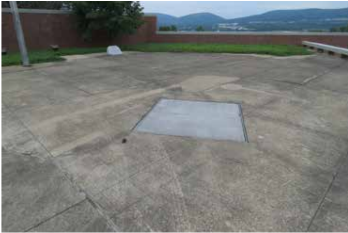
Water valve vault to remain
