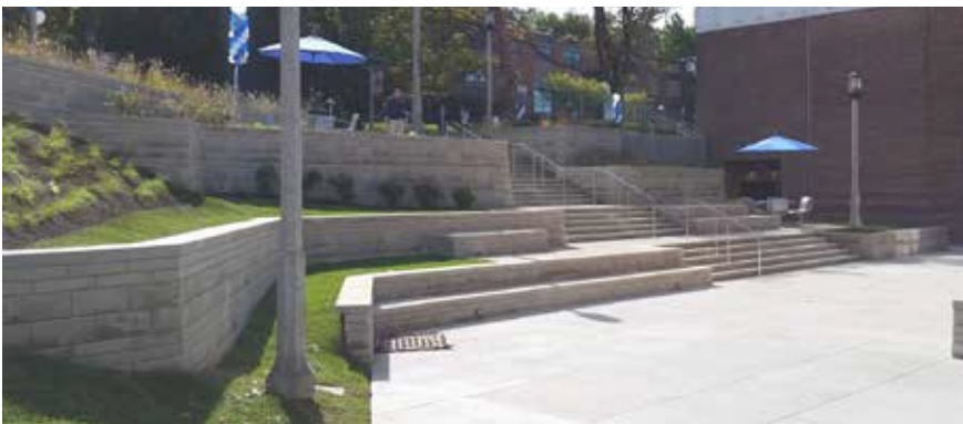
York Ruhl Center retaining wall system - example of potential wall redesign
