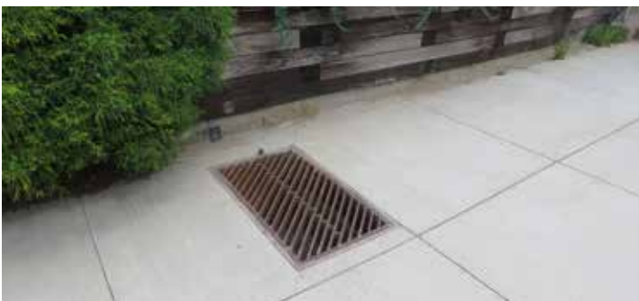
3. Avoid large inlets in pavement and ensure grates are safe
