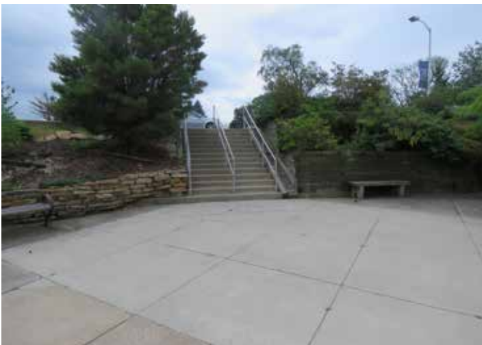
Steep steps with no landings & mismatched retaining walls
