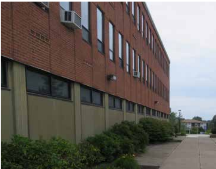
Old style wall-mounted lights (wall packs) at Dawson
