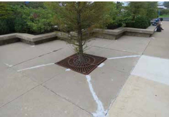
Tree pits unnecessary and stunt tree growth
