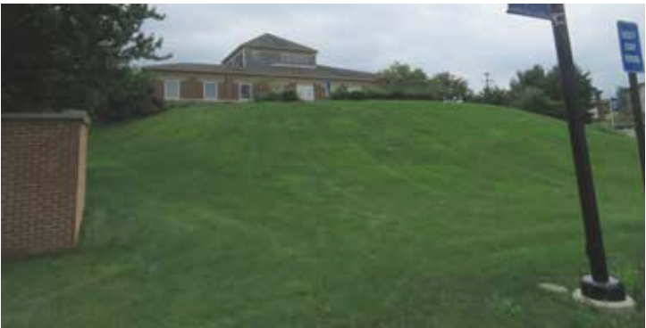
Large embankments are stark and imposing
