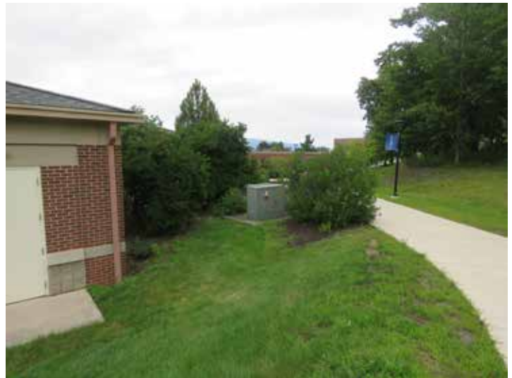
Gaps in screen plantings in a couple locations reveal utilities
