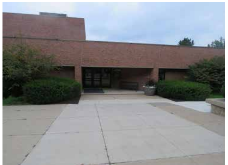
Excessive, patched pavement and tired landscaping
