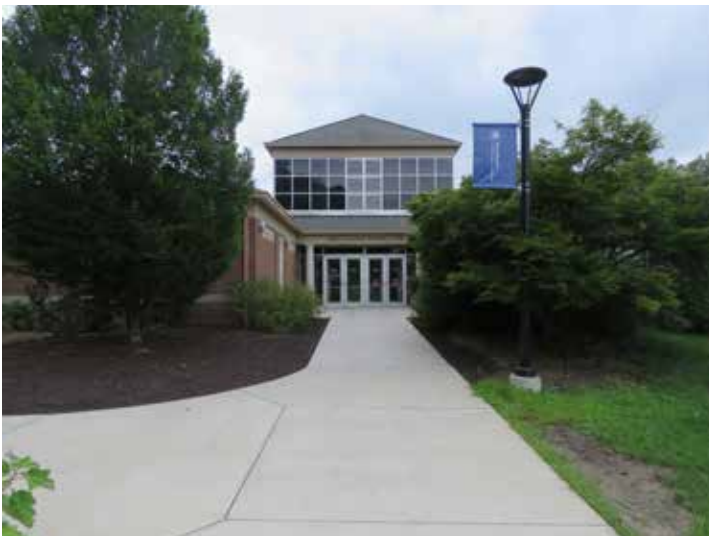
Missing plants on left side & overgrown plants on right side
