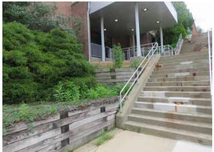
Close up of mid-level entrance from below
