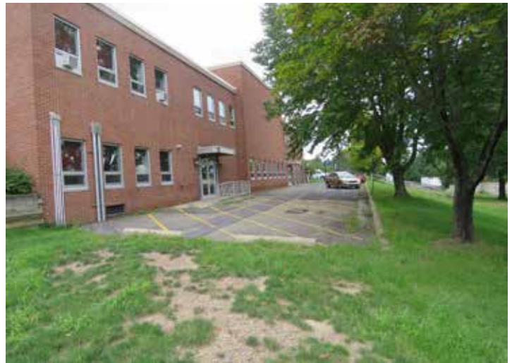
Parking, access drive, & building entrance are in disrepair
