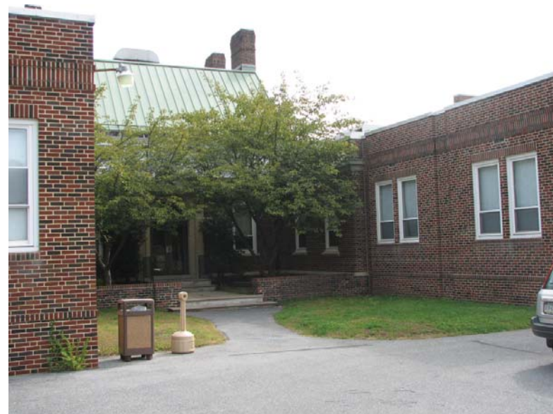
Existing main west entrance from parking lot
