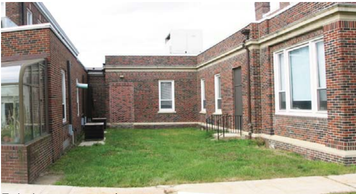
Existing secondary entrance on east side of building
