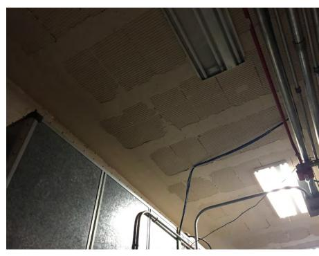
Ribbed Clay Tile Fillers Shown in Between Smooth Concrete Beams
