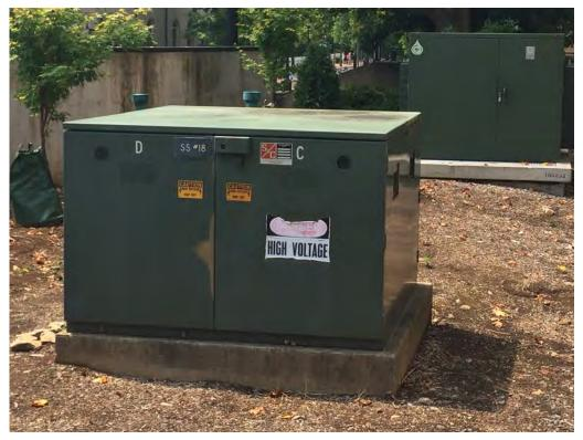
Medium Voltage Switch and Building Transformer
