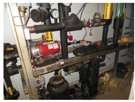
Secondary Chilled Water Pump Loop with Plate and Frame Heat Exchanger
