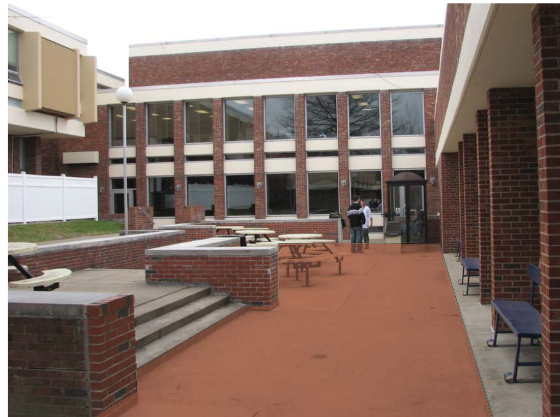
Resurface and level without removal of existing surface and drainage.
